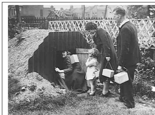
A typical Anderson shelter. Note the gas masks, being carried in the issue cardboard boxes..
